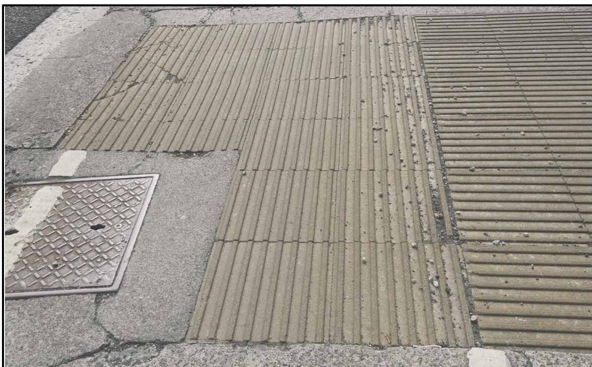
Figure 3.14: Broken Tactile Paving at Shared Surface
